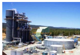
Natural Gas Fired Co-generation Plants
