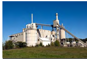
Coal, Biomass Fired Thermal Power & Co-generation Plants
